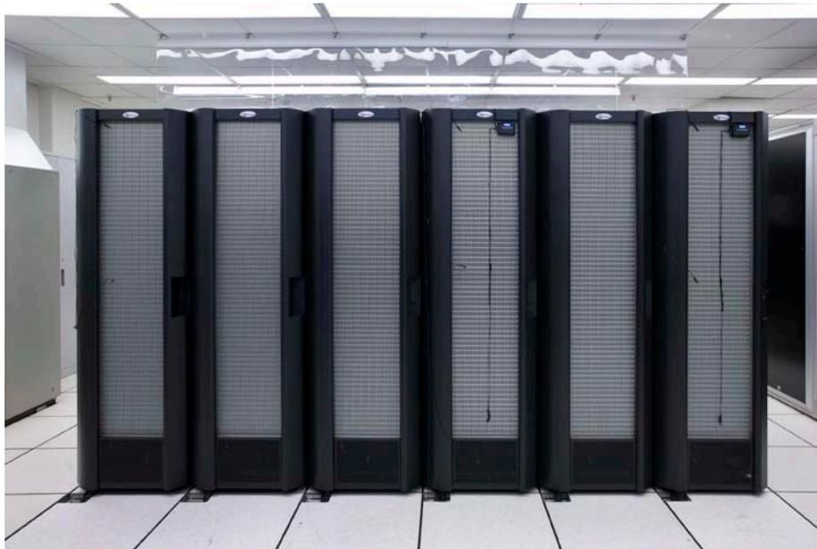
**Figure 1: Passive Rear Door Heat Exchanger devices at LBNL**
