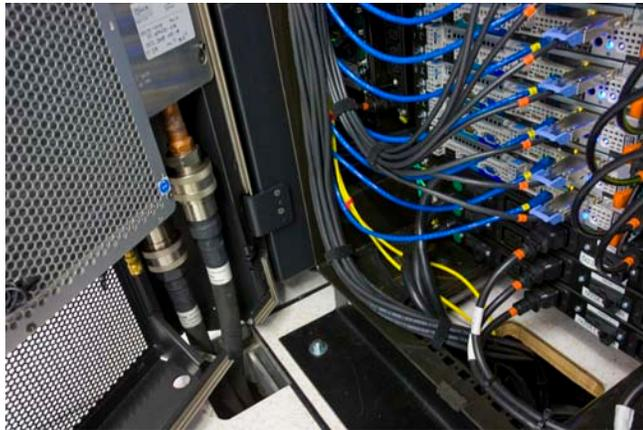
**Figure2: RDHx hose connections**
